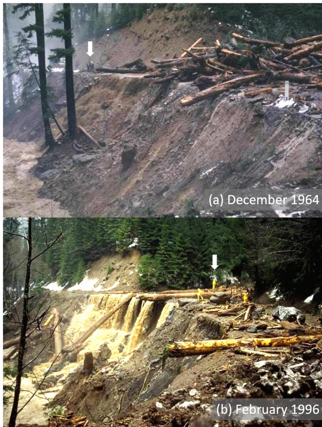
FIGURE 5 Photographs of debris flow deposits on the road passing by the mouth of the Watershed 3 stream (entering from the upper right) where it reaches Lookout Creek (lower left) (see location in Figure 4). (a) Pile of large wood delivered by the third pulse of multiple debris flows from watershed 3 on the night of 22–23 December 1964. Two previous pulses occurred during the night and early morning of 21–22 December (Fredriksen, 1965). Thirty-two landslides moved an estimated 30 000 m 3 of sediment (300 m 3 /ha) in the watershed. Twenty-nine of the 32 landslides were adjacent to stream channels, and 93% of the material originated from road-related slides (Fredriksen, 1970). (b) Deposit from debris flows on the night of 6–7 February 1996 showing fewer very large wood pieces in 1996 compared to 1964. Note human figures for scale indicated by white arrows. Photo credits: 1964, Dick Fredriksen; 1996, Al Levno.
